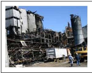
OSHA Currently. recommends following the NFPA 654, Standard for the Prevention of Fire and Dust Explosions from the Manufacturing, Processing, and Handling of Combustible Particulate Solids. This standard requires the use of an approved explosion proof vacuums that meet UL standards Class I, Div 1 and 2, Group D and Class II, Div 1 and 2, Group F & G.
